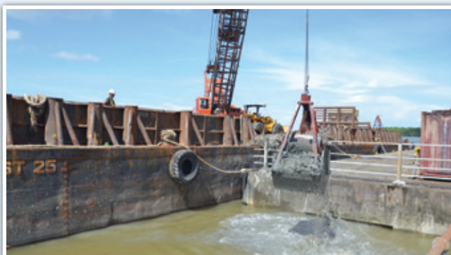
Penyelenggaraan pengerukan dermaga di Terminal Senari dan Pending. Maintenance dredging alongside wharves at Senari and Pending Terminal.
