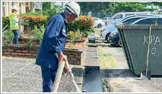
Pembersihan longkang bagi mengelakkan pembiakan nyamuk AEDES di Terminal Pending. Flushing of drain to prevent AEDES mosquito breeding at Pending Terminal.
