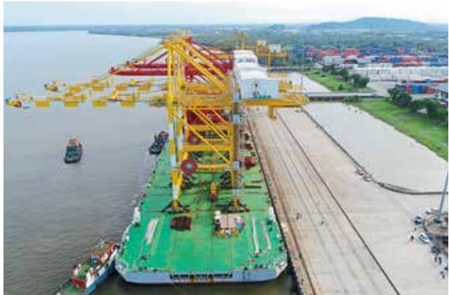
Two new quay cranes (yellow) being skidded onto the wharf of Senari Terminal
